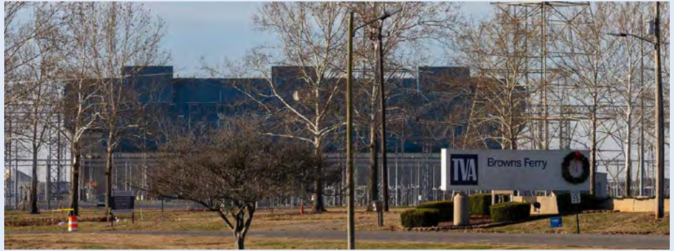
Browns Ferry Nuclear Plant
