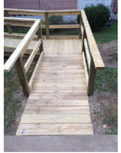
The Swafford ramp completed by the Cleveland Chapter
