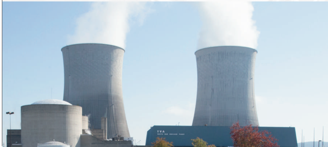
Watts Bar Nuclear Plant
