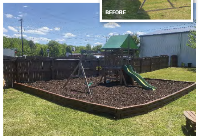
The completed project
