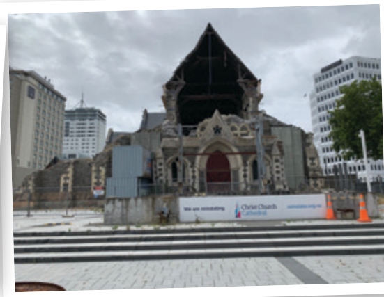
Christ Church Cathedral, built in the 1800s, is still under repair from 2010-2011 earthquakes, in Christchurch, New Zealand.
