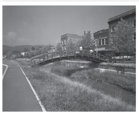
Bridges and walkway — results of Townlift work at Coeburn, Va. Teams of TVA planners, architects, and engineers “helped local people decide what they wanted to do with their downtown . . . people really appreciated this kind of assistance from TVA.” — Interview with John Cartwright, June 18, 2018
