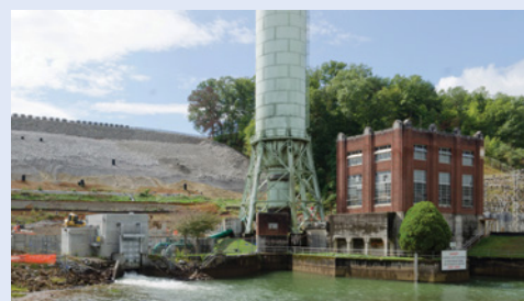
Blue Ridge Dam
