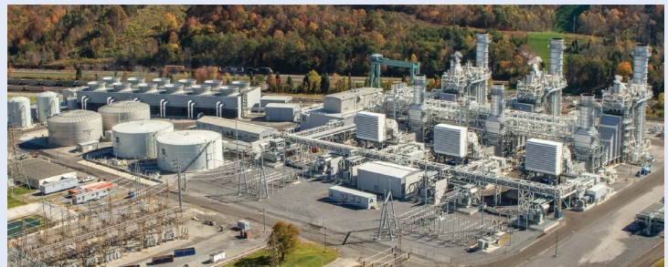
John Sevier Combined Cycle Gas Plant
