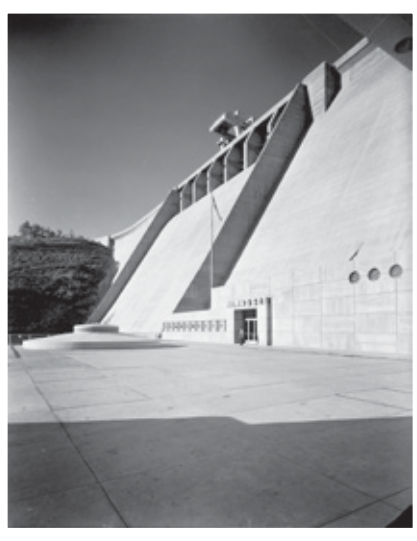
Hiwassee Dam and Powerhouse, October 1940
