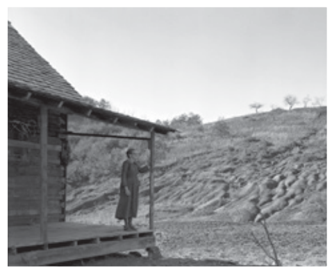
Erosion at House on Sevierville Pike, February 1939
