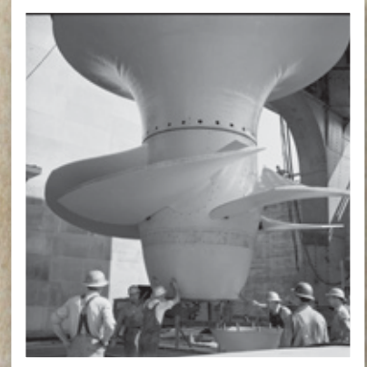
Turbines at Fort Loudoun Dam, August 1943
