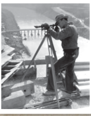
Engineer silhouette, during construction on Norris Dam, May 1935
