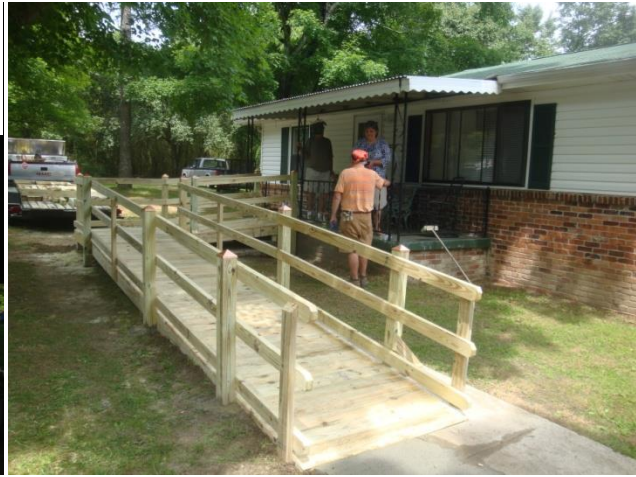
Completed ramp May 29, 2014
