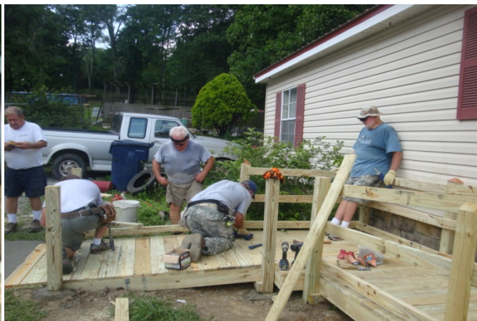
Installation of ramp
