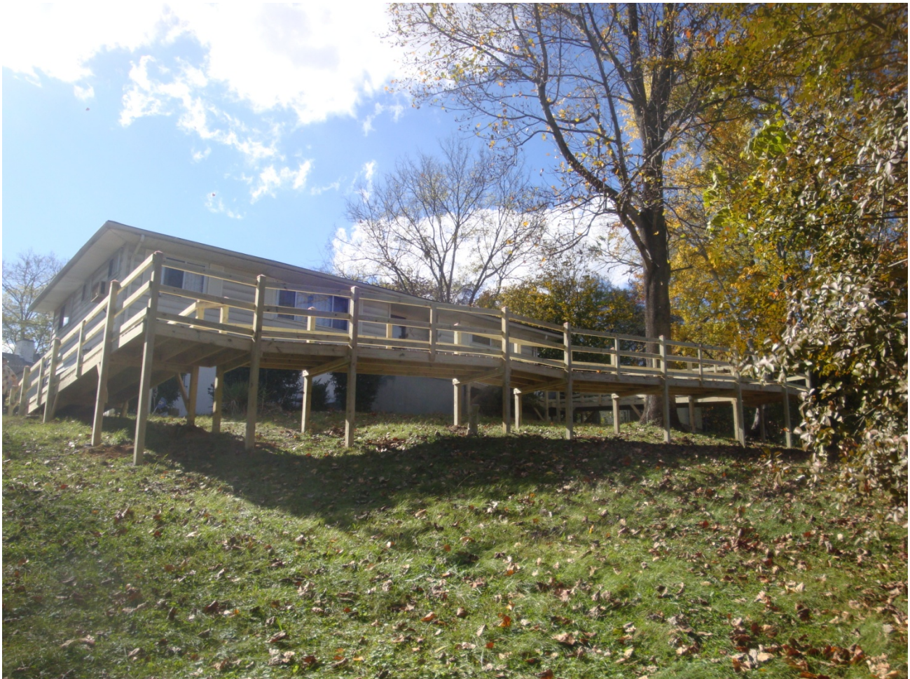
Completed Ramp ~199 linear feet
